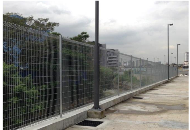
Anti Climb Perimeter Fencing
